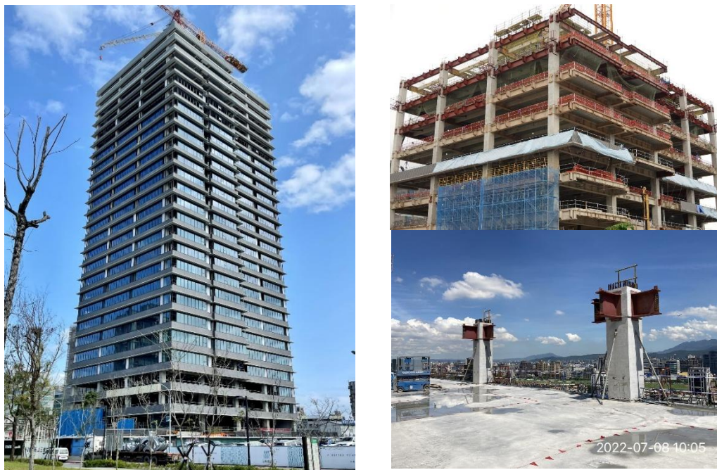
Fig. 42: View of the whole building and the typical steel-concrete MRCF connection detail.
